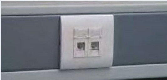
• Socket for data transfer / Telephone
